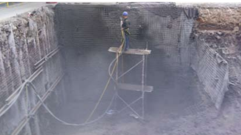
Application of shotcrete
