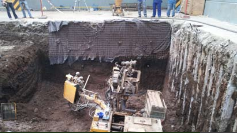
Installation of the anchors and the excavation of the soil
