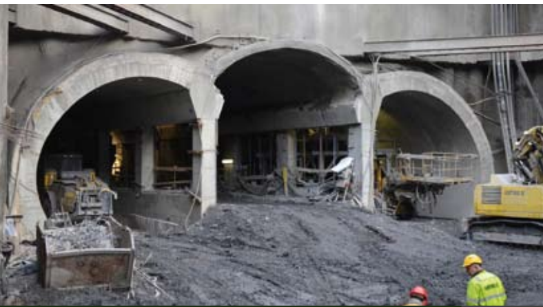
Portal of the mined triple-span metro station
