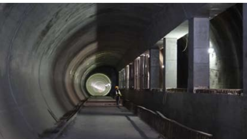
Completed final lining of a side station tunnel
