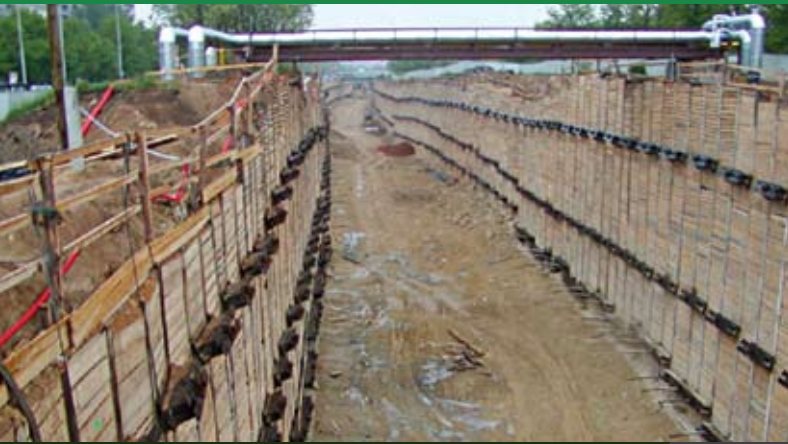
Open pit for the cut-and-cover tunnels between the Střížkov and Prosek stations
