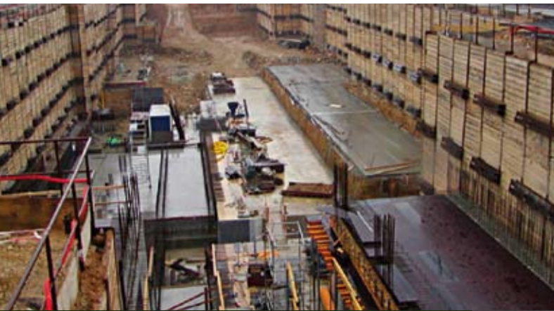
Prosek station - open pit
